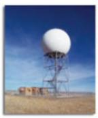
Air radar used to identify powerful storms and track their movements.
