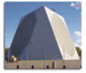
This 27-meter-high radar facility, reminiscent of a fly's eye, scans the sky above northern Alaska and is used as an early warning system against ballistic missiles.
