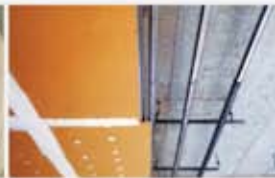
GYPSUM BOARD CEILING
